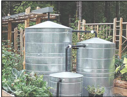
Water will be collected in containers from areas around the site including the false roof, the rain garden, and the bioswale.
